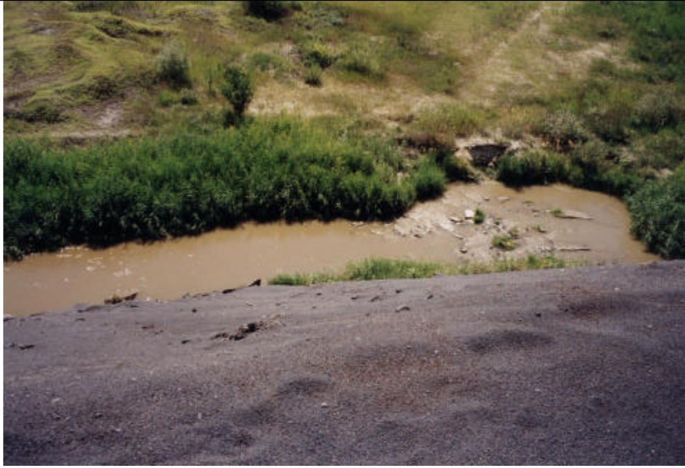
**Photo 11: Rain Water will wash Slope Material directly into Tarnava River**
