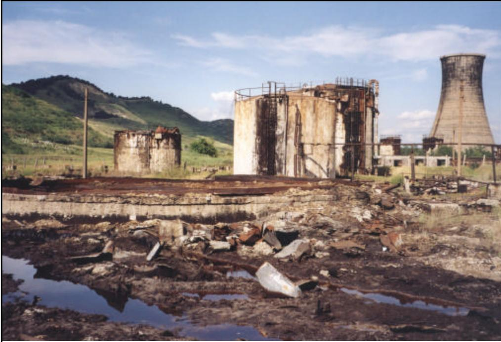
**Photo 11: Soil Contamination nearby Storage Tanks**
